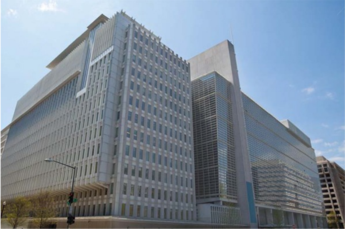
The North Side Headquarters for the World Bank in Washington DC.
